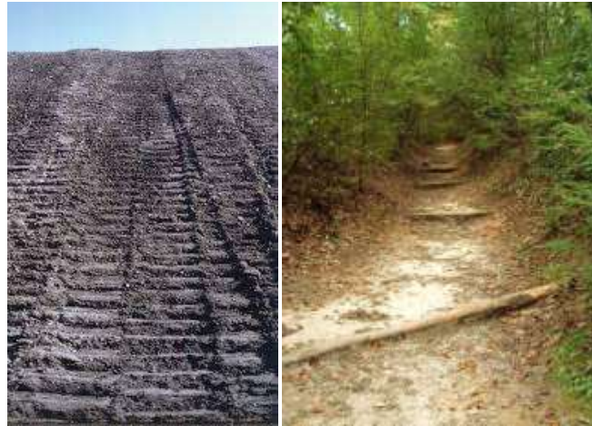
Figure 9. Rough grading (left) and waterbars (right).
