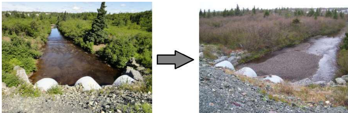
Figure 5. Changes in river morphology due to sedimentation.
