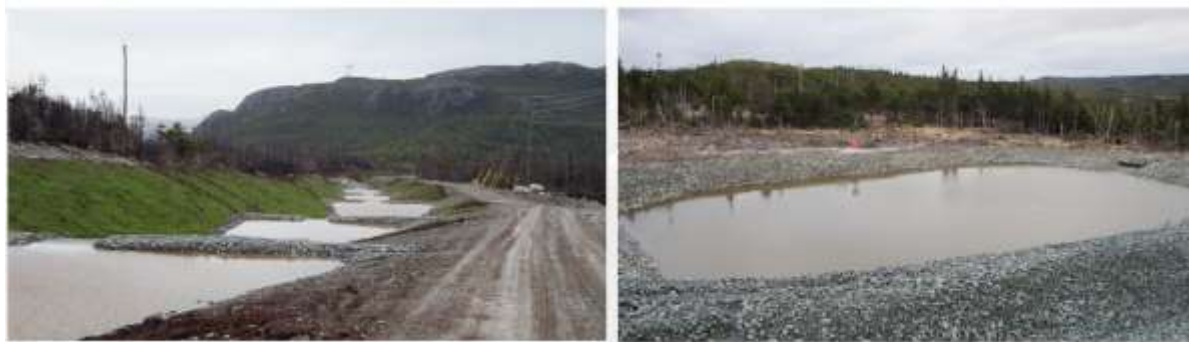
Figure 12. Settling pools within a diversion ditch (left), settling pond (right).
